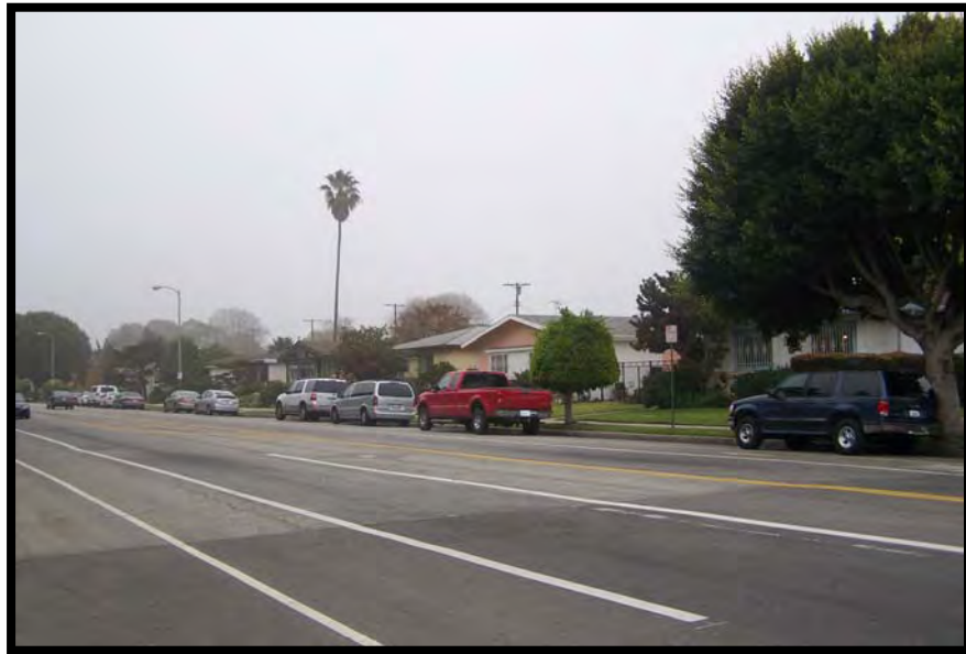
Photo A2. View to southeast from north side of Rose Avenue and Frederick Street. Notice the late-historic period Ranch style homes (Penmar Project Area).
