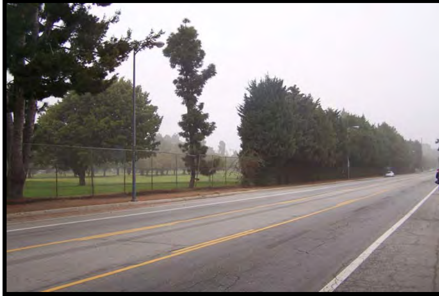
Photo A5. View to east-northeast from south side of Rose Avenue at Courtland Street, along proposed trench for force main (3) conduits in north half of Rose Avenue. Penmar Municipal Golf Course in background (Penmar Project Area).
