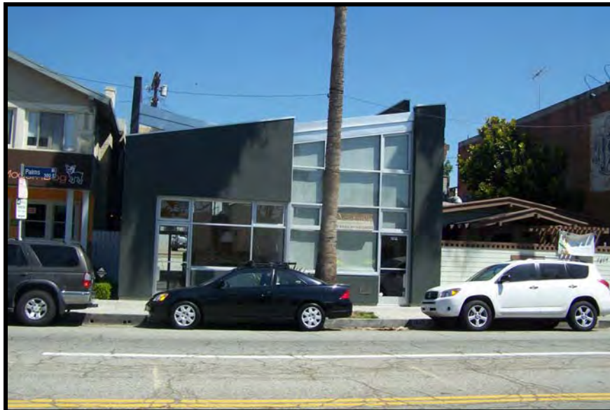
Photo A38. View to north side of Abbot Kinney Boulevard, southeast of intersection of Palms Boulevard (Abbot Kinney Boulevard Project Area).
