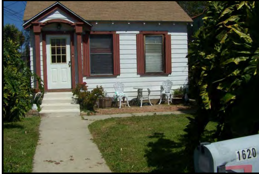
Photo A24. 1620 Crescent Place, north side of pedestrian paved trail (Rialto Court/Crescent Place Project Area).
