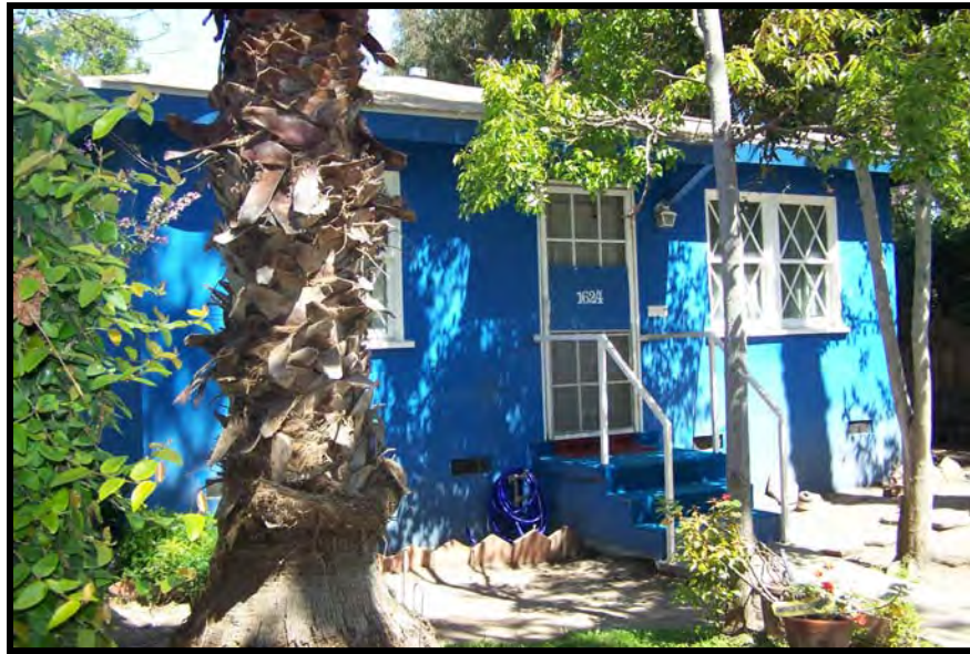
Photo A28. 1624 Crescent Place, north side of the paved pedestrian trail (Rialto Court/Crescent Place Project Area).
