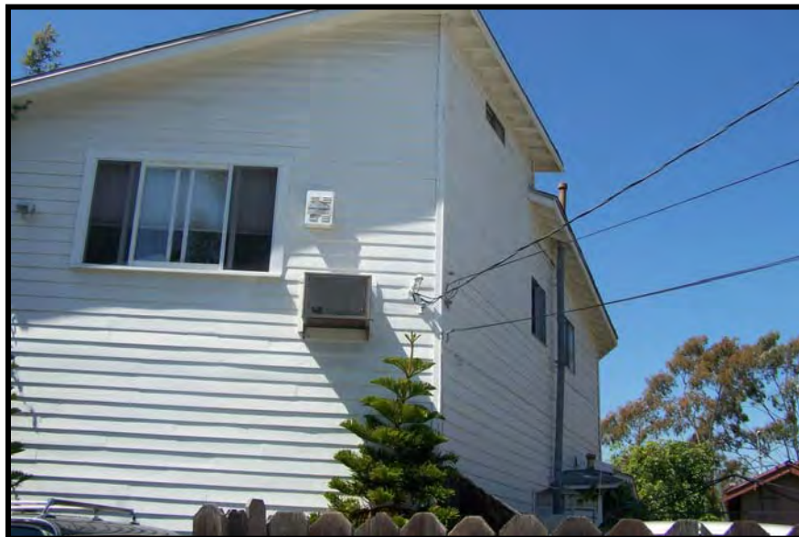
Photo A33. Rear of 1614 Crescent Place from Rialto Court (Rialto Court/Crescent Place Project Area).
