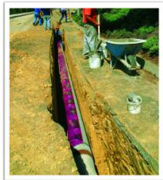
Installation of recycled water pipeline.
