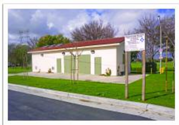
Hollydale Pump Station at Hollydale Park in the city of South Gate.
